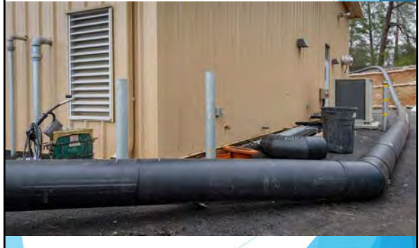
Testing High-Lift Pumps
