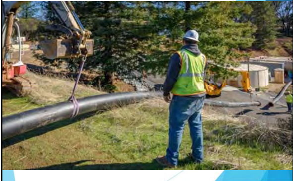
Raw Water to Old Plant
