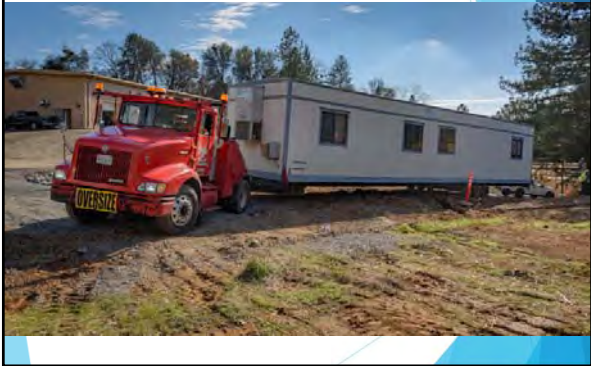
Removing Construction Office Trailer
