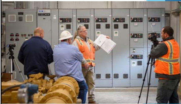
Training in the Raw Water Pump Station
