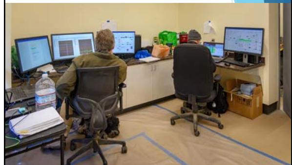
Westech and KBL Working on Filter Controls
