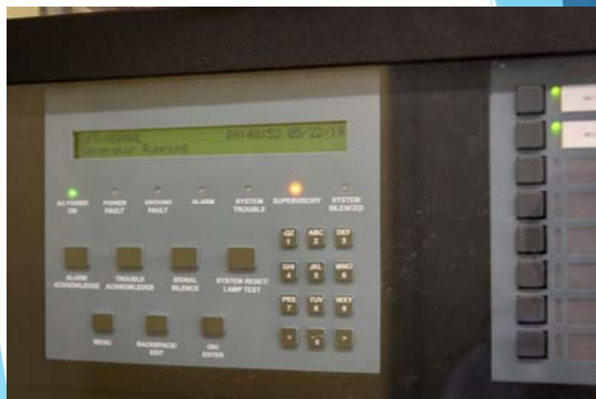
Generator Operation During Planned Power Outage
