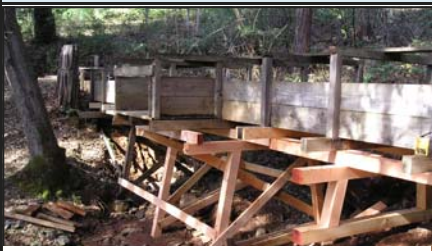
Repaired flume
