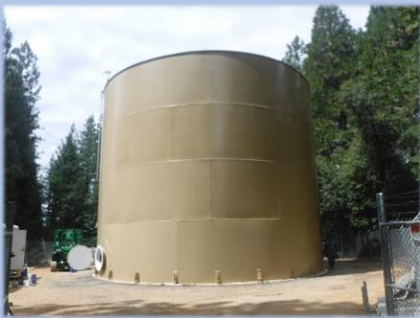
Walton Lake Storage Tank #2
