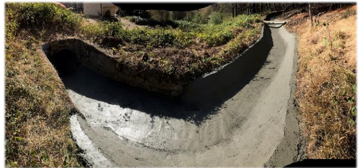
Lined Section of Ditch
