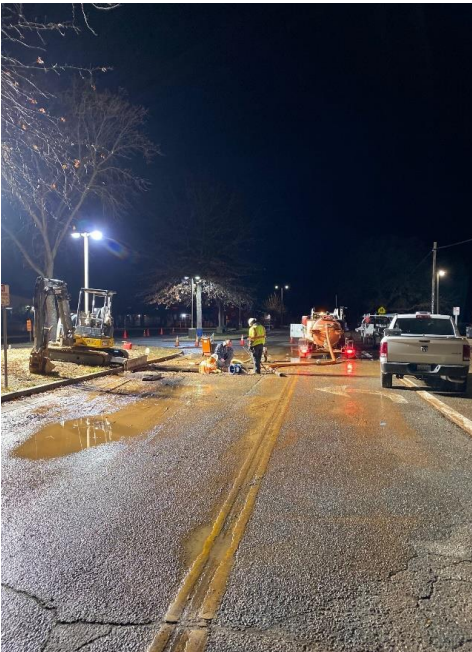
District crew repairing a break near Northside School.
