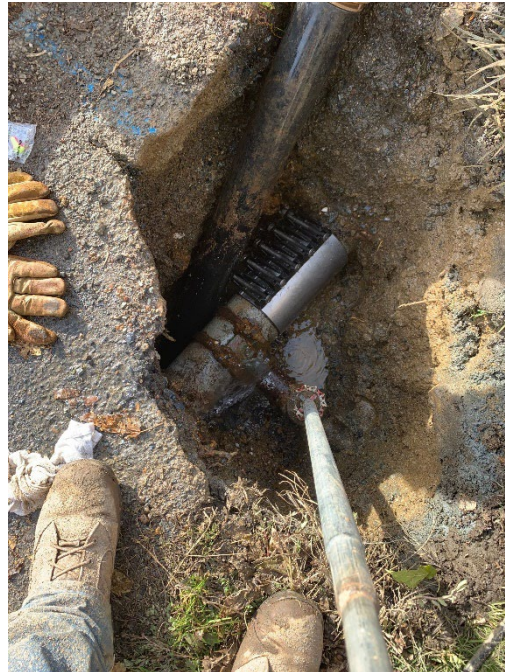
Main Break Task – | 9 Labor Hours | Vac Trailer, Service/Dump Truck, Hand Tools
