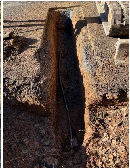
Service Line Replacement – 22 Labor Hours | Dump/Service Truck, Vac Trailer, Hand Tools, Mini-Excavator
