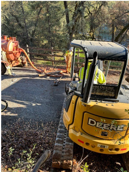
Service Line Replacement – 22 Labor Hours | Dump/Service Truck, Vac Trailer, Hand Tools, Mini-Excavator
