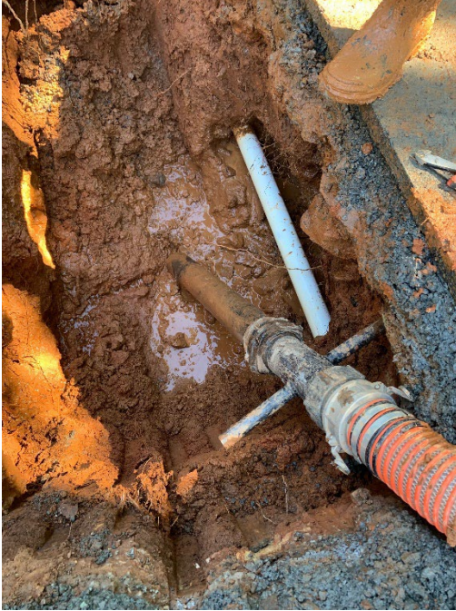
Main Line Break – 21 Labor Hours | Dump Truck, Vac Trailer, Excavator, Service Trucks, Hand Tools, Line Detector, Loader
