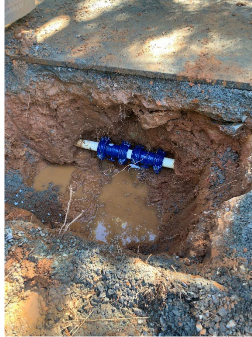
Main Line Break – 21 Labor Hours | Dump Truck, Vac Trailer, Excavator, Service Trucks, Hand Tools, Line Detector, Loader
