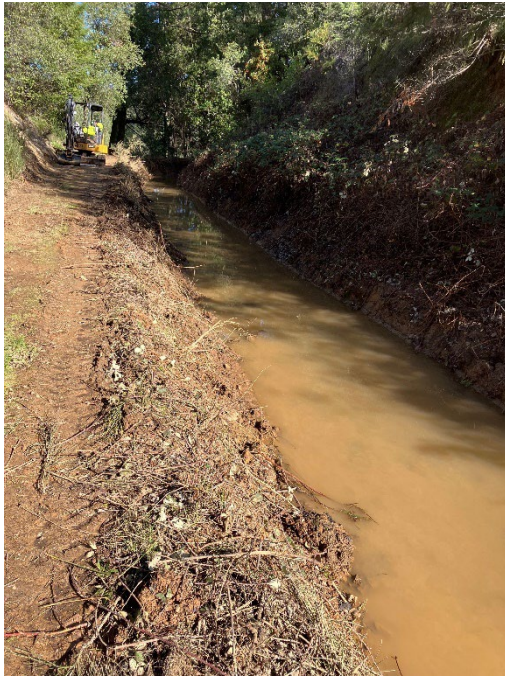
Main Ditch Vegetation Clearing – 16 Labor Hours | Excavator, Service Truck
