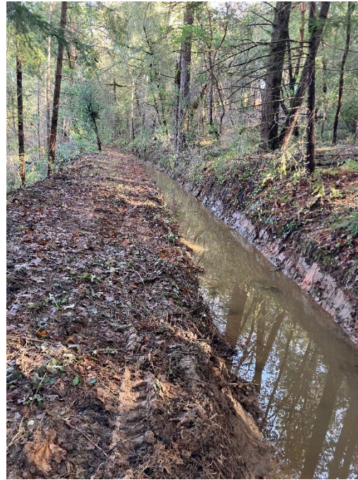
Main Ditch Vegetation Clearing – 16 Labor Hours | Excavator, Service Truck
