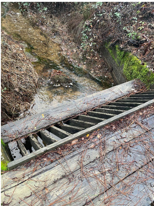
Trillium Vegetation Rack Rehabilitation – 38 Labor Hours | Metal/Lumber, Welder, Hand Tools
