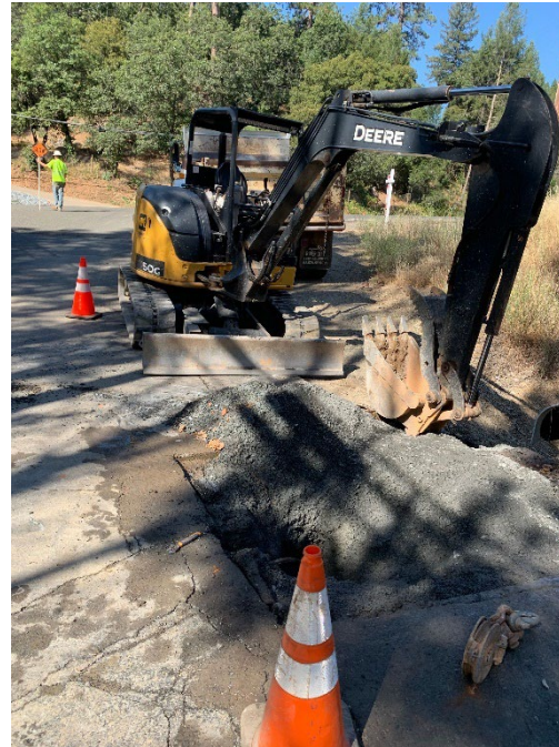
Service Line Replacement – 35 Labor Hours | Dump Truck, Vac Trailer, Excavator, Service Trucks, Hand Tools
