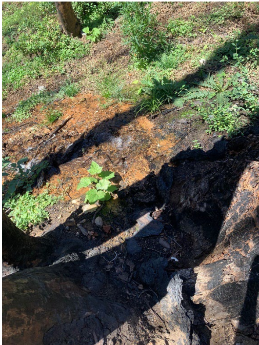
Upper Canal Break – ~One CFS | 26 Labor Hours | Mini-Excavator, Dump Truck, Service Trucks, Rock/Plug
