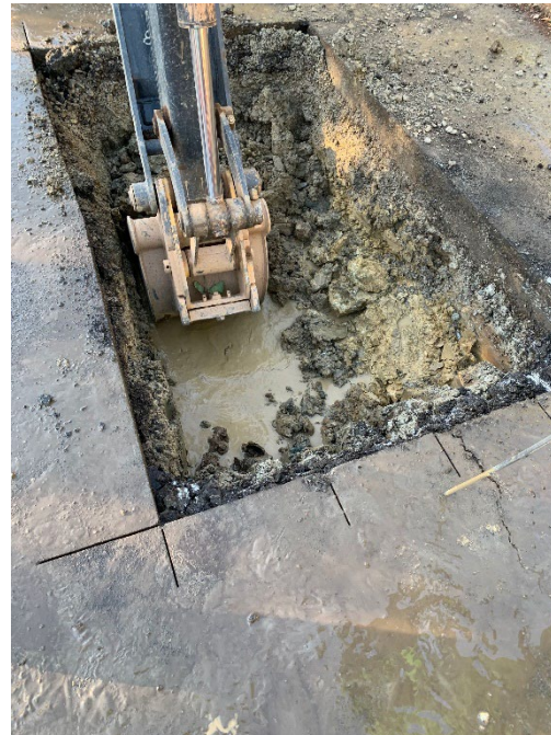
Hydrant Repair and Main Break
