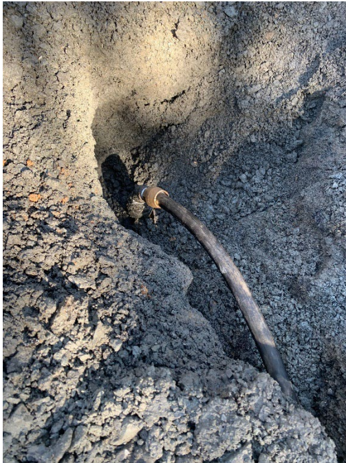
Service Line Replacement – 35 Labor Hours | Dump Truck, Vac Trailer, Excavator, Service Trucks, Hand Tools
