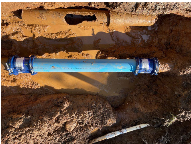
Garden Valley Pipeline Repair – 18 Labor Hours | Excavator, Dump/Utility Truck
