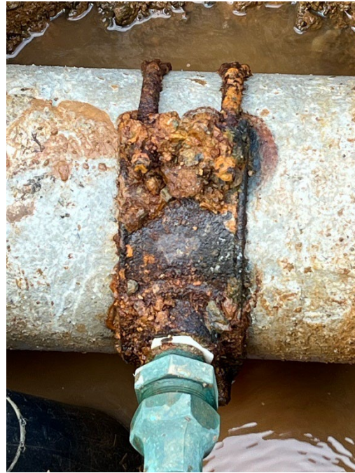
Main Saddle/Later Repair – 30 Labor Hours | Excavator, Vacuum Trailer, Service/Dump Truck, Hand Tools
