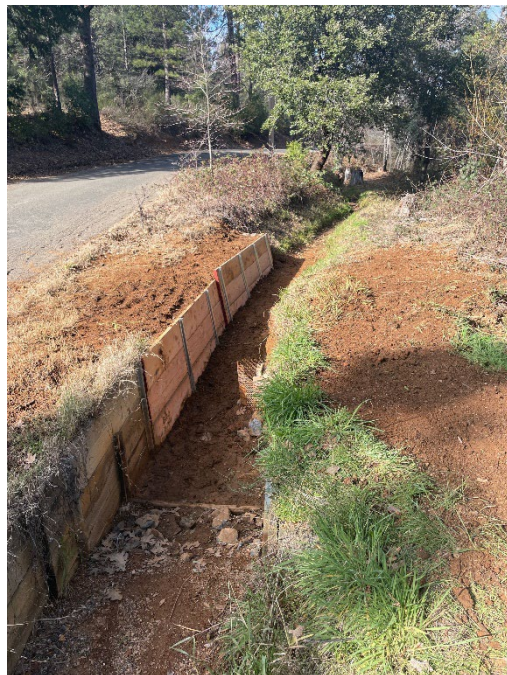
Taylor Mine Ditch Crib Wall Improvement – 28 Labor Hours | Utility Trucks, Hand Tools
