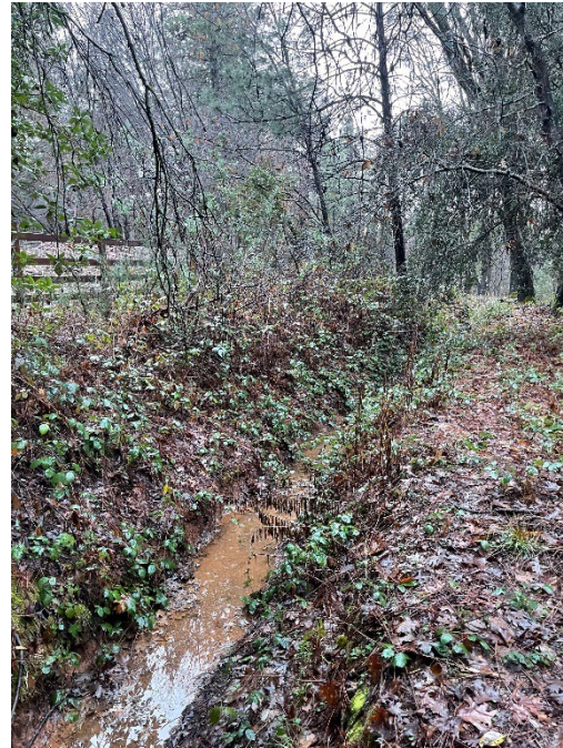
Kelsey Ditch Cleaning – 920 Feet | 34 Labor Hours | Excavator, Service Truck
