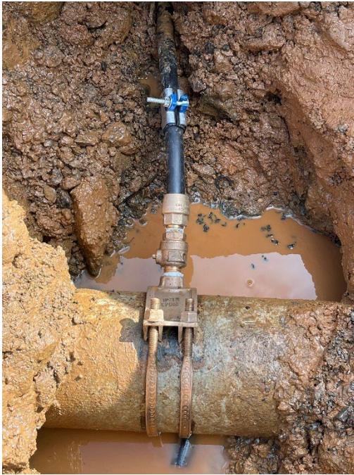
Main Saddle/Later Repair – 30 Labor Hours | Excavator, Vacuum Trailer, Service/Dump Truck, Hand Tools
